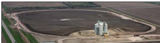
Higher-altitude photo shows the facility's nearly 9,000-foot loop track and its switch with a Burlington Northern Santa Fe main line.
