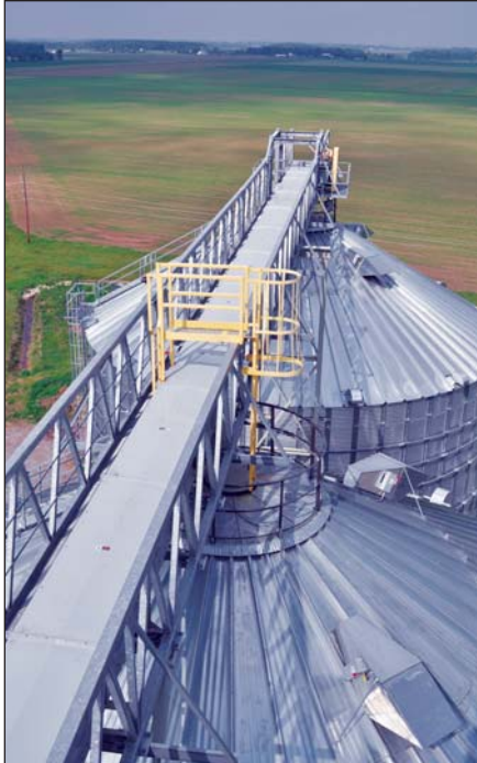
West Findlay's new Behlen tanks are fed by 30,000-bph GSI drag conveyors.
