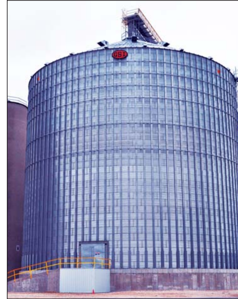
Blanchard Valley's new 730,000 bushel GSI corrugated steel tank in Fostoria.
