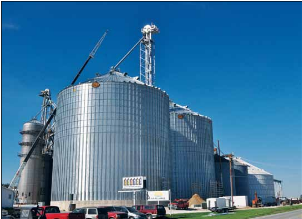
Co-Alliance LLP's 4.1-million-bushel elevator near Goodland, IN, with two new 750,000-bushel GSI corrugated steel tanks in foreground. Photos by Ed Zdrojewski.
