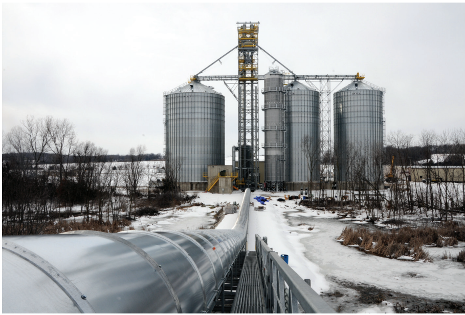
The barge-loading conveyor is 1,136 feet in length and served by a 36-inch, single-piece, rubber belt conveyor. Grain is conveyed at 30,000 bph, with barges loaded in less than three hours.
