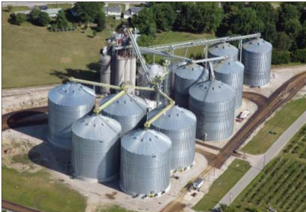
Sunrise Cooperative's huge 6.5-million-bushel rail loading complex in Clyde, OH. The two newest tanks, holding 738,000 bushels each, are in the foreground. Aerial photo by Focal Plane Photography LLC, South Euclid, OH.
