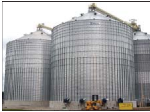
Closeup view of the two newest tanks at Clyde, Behlen models standing 105 feet in diameter and approximately 89 feet tall at the eaves. Photo by Ed Zdrojewski.
