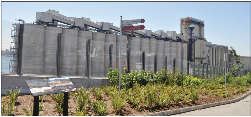
New annex at the North Vancouver terminal as viewed from a municipal walking trail on a bluff overlooking the harbor.
