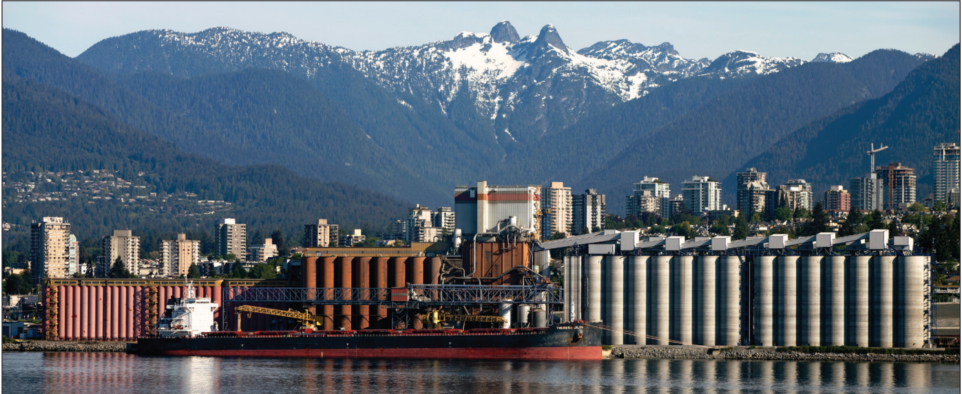
Richardson International's export terminal in North Vancouver, BC, Canada. New 80,000-metric-tonne slipform concrete annex is the gray section at right. Photo courtesy of Richardson International.
