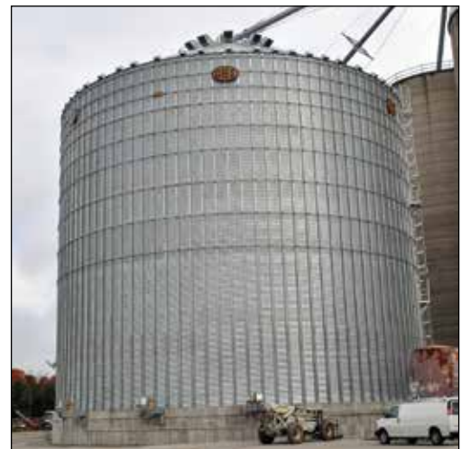
Closeup of the new GSI corrugated steel tank.
