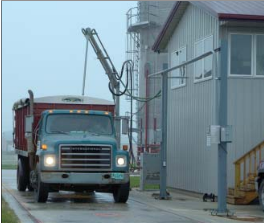
Incoming grain is weighed on a Thurman pit-type scale while being sampled with an InterSystems truck probe. The same scale will be utilized later to determine tare weight.
