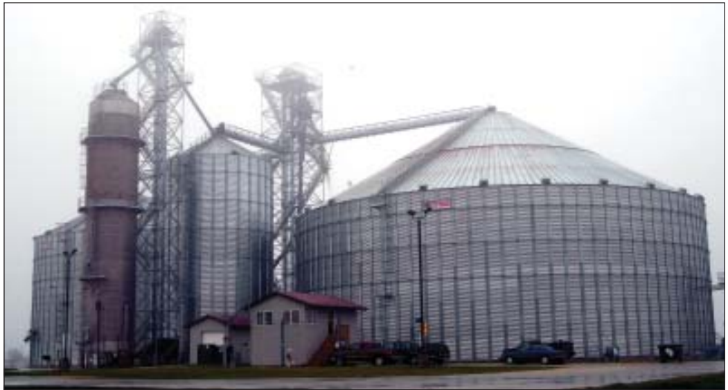
Olsen's Mill Inc.'s new 1.6-million-bushel grain elevator at Viroqua, WI on a foggy fall morning. Photos by Ed Zdrojewski.
