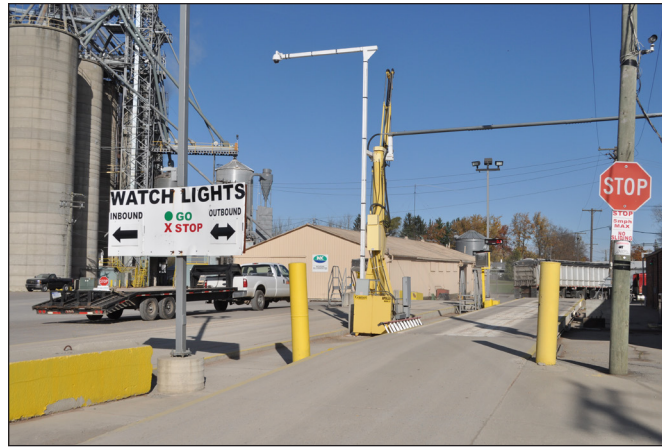
New outbound truck scale and truck probe at Marlette.
