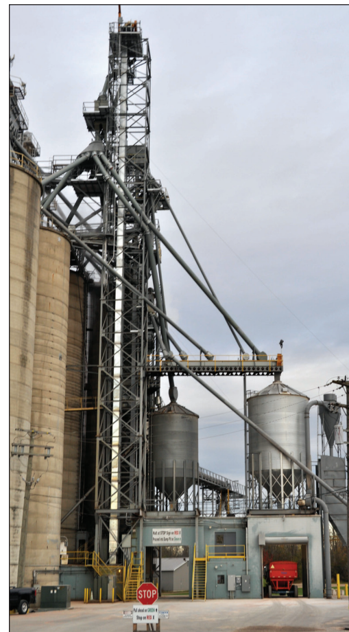
Closeup of new leg and receiving pit (far right) at Marlette.
