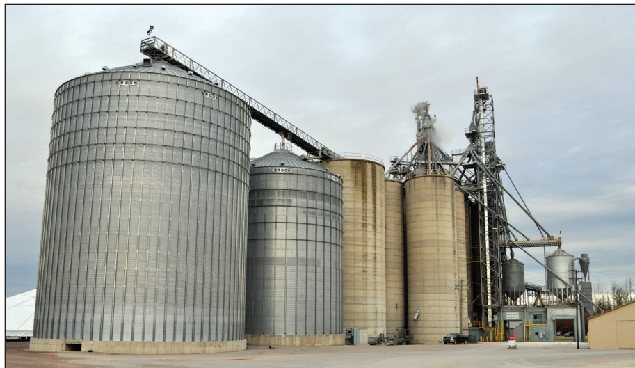
Elevator at Marlette, MI, with new 20,000-bph leg and receiving pit at far right.
