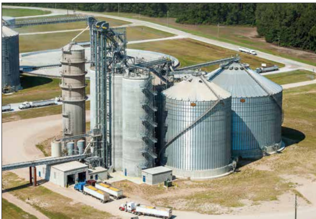
Louis Dreyfus Commodities' new river terminal in Rosedale, MS, featuring 2.2 million bushels of upright storage and 40,000-bph throughput speed. Aerial photos by Rory Doyle, Cleveland, MS.
