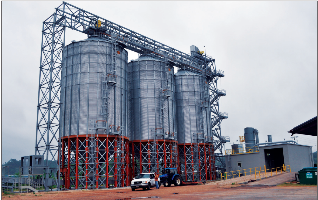
Steel storage and truck receiving pit at Louis Dreyfus Commodities' new 120,000-bushel barge terminal on the Mississippi River in Natchez, MS. Photos by Ed Zdrojewski.
