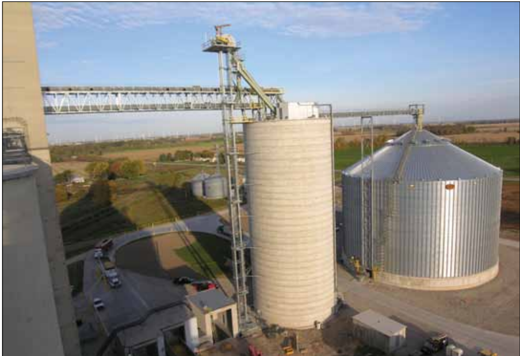
New construction at Cooperative Elevator Co. in Elkton, MI includes, from left, a third receiving pit, 30,000-bph GSI receiving leg, 285,000-bushel Hoffmann jumpform concrete silo, and a 1-million-bushel GSI corrugated steel tank. Photos courtesy of Elevator Services & Storage, Inc., Portrait photo by In Focus Photography, Pigeon, MI.
