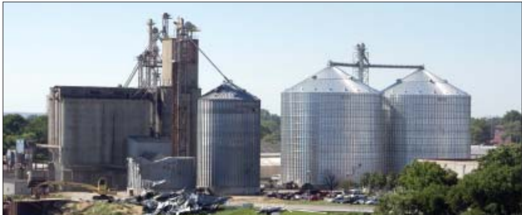
Alabama Farmers Cooperative's river terminal at Decatur, AL, with new 1.5-million-bushel steel annex at right, viewed from the nearby U.S. Highway 31 bridge over the Tennessee River. Photos by Ed Zdrojewski.
