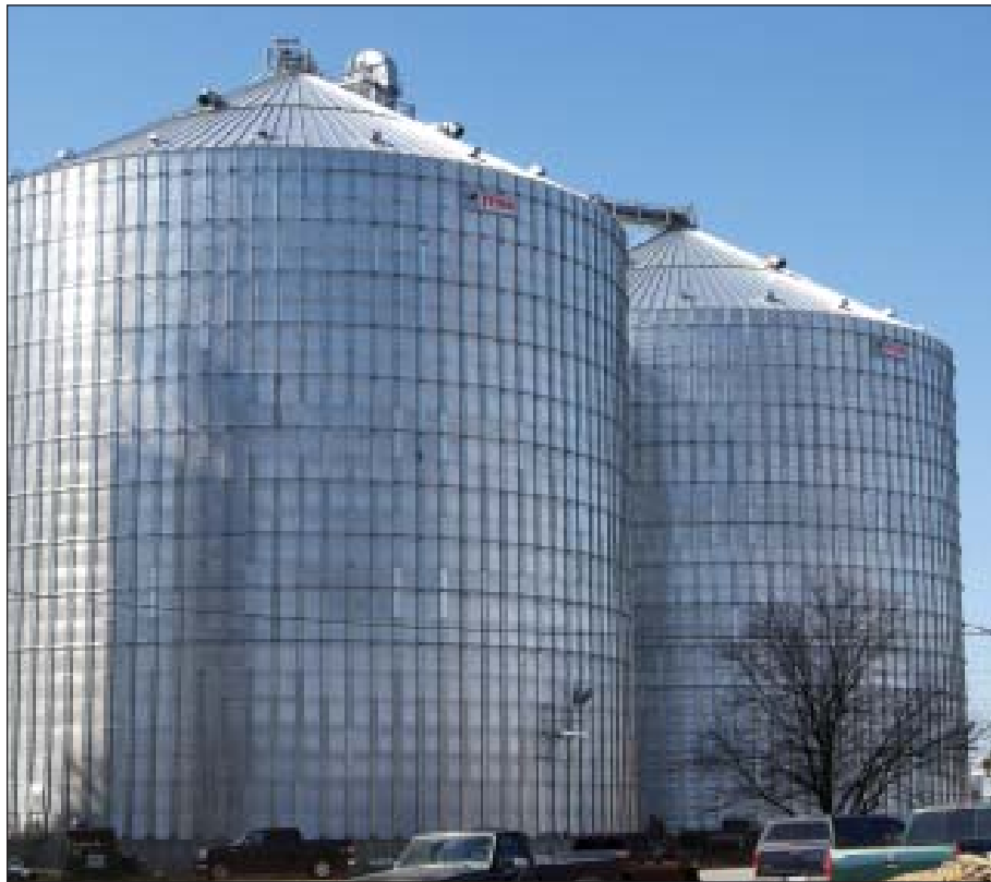
Closeup of two new 750,000-bushel Chief Titan corrugated steel tanks making up the annex.
