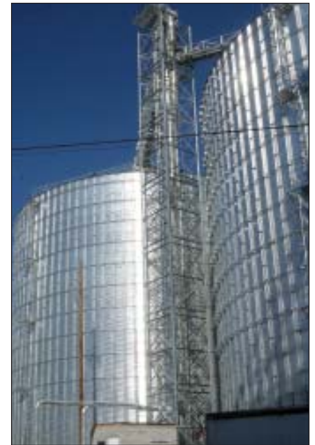
New 18,000-bph Chief receiving leg serving the annex, which empties onto a pair of overhead Hi Roller enclosed belt conveyors.
