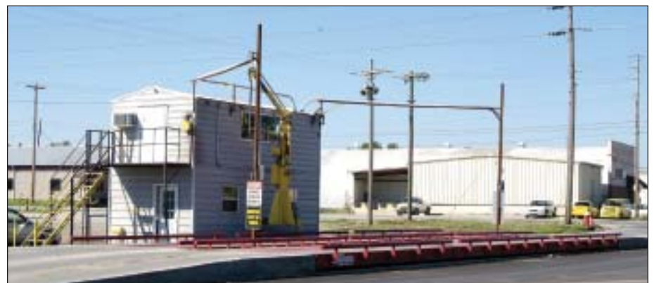
New two-story scalehouse features inbound and outbound Rice Lake truck scales and an Apollo truck probe.
