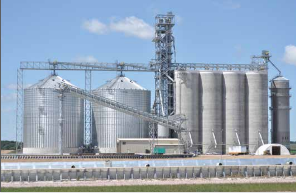
New 81-20 Grain LLC rail-loading terminal near Randolph, NE holds 4.5 million bushels of grain in a combination of concrete, steel, and temporary storage.
