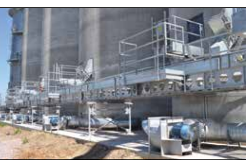
Four slipform concrete wet tanks empty onto a 15,000-bph InterSystems above-ground conveyor running out to a 10,000-bph Zimmerman dryer. The tanks are equipped with an AIRLANCO Airauger aeration/unloading system.
