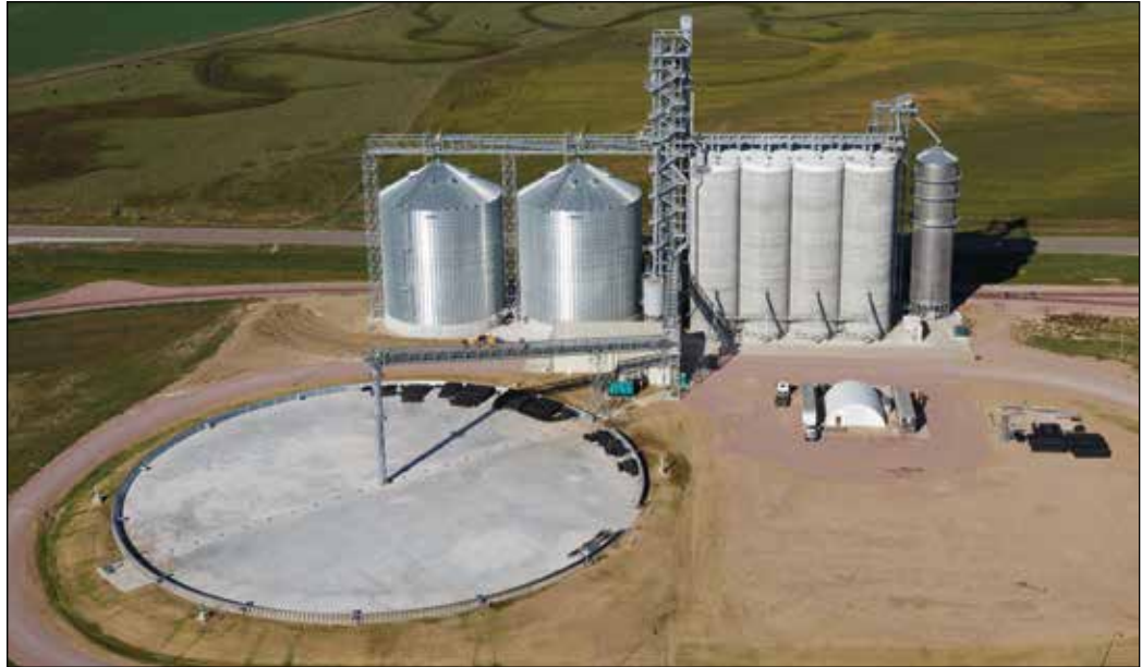
New 81-20 Grain LLC rail-loading terminal near Randolph, NE holds 4.5 million bushels of grain in a combination of concrete, steel, and temporary storage. Aerial photo by Kansas Aerial Photography, Minneapolis, KS.
