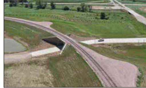
The entrance driveway into the 81-20 Grain terminal runs underneath the facility's loop track. In the distance is the highway intersection for which the joint venture is named.
