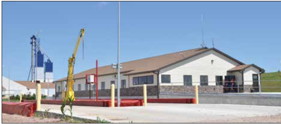
Rice Lake 80-foot pitless inbound and outbound scales are located adjacent to the facility office, where trucks are sampled with an Apollo probe.
