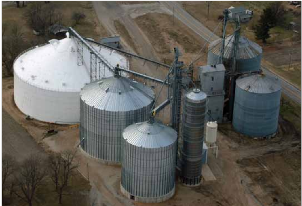
Farmers Grain & Coal Co.'s branch elevator at Teheran, IL, with two new Behlen steel tanks, Brock dryer, and Union Iron legs in foreground. Aerial photo by Steve Huey, Pekin, IL.
