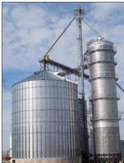
Ground level view of new Behlen wet and dry tanks and 7,000-bph Brock tower dryer. Photo by Ed Zdrojewski.
