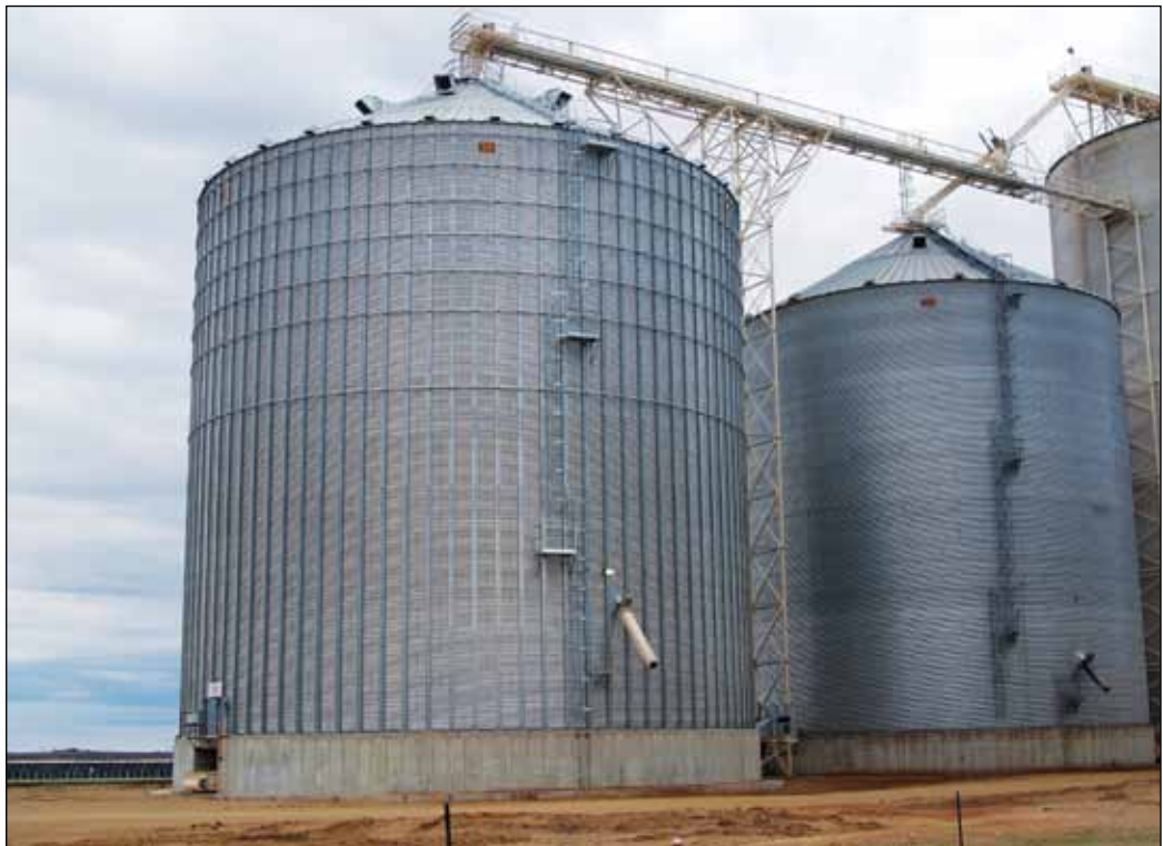
Closeup of the new GSI 500,000-bushel tank at Madison showing sidedraw and overhead 20,000-bph Hi Roller enclosed belt conveyor. Photos by Ed Zdrojewski.
