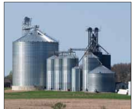
Overall shot of the branch elevator at Ramona.
