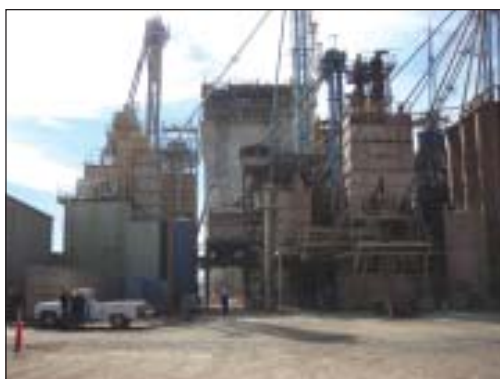
The old Eagle Milling feed mill on the Casa Grande site was entirely open air, made possible by a warm desert climate. Photo courtesy of Cargill Animal Nutrition.
